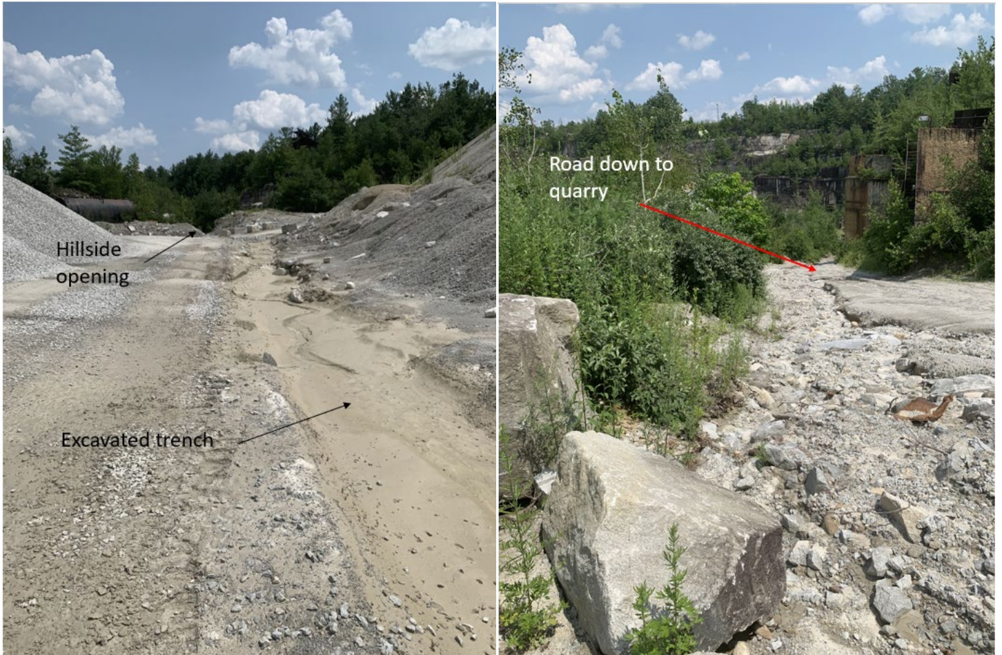
Figure 5: June 12, 2023, Site Visit Photos of Drainage Path from Rock Crushing Area Pond
