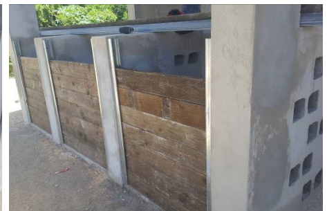
The Iguels collect and store the wood-chip waste in the piggery's block-bin storage facility for later use as compost for plants.
