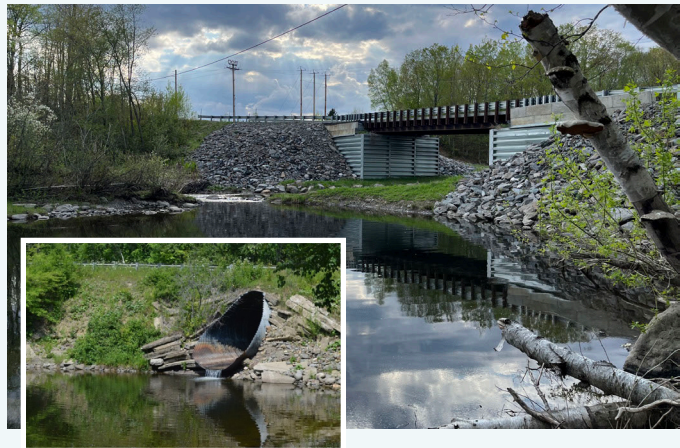
HBMI and its partners replaced the perched culvert (inset photo) on Moose Brook with a bridge that allows unrestricted fish passage.
