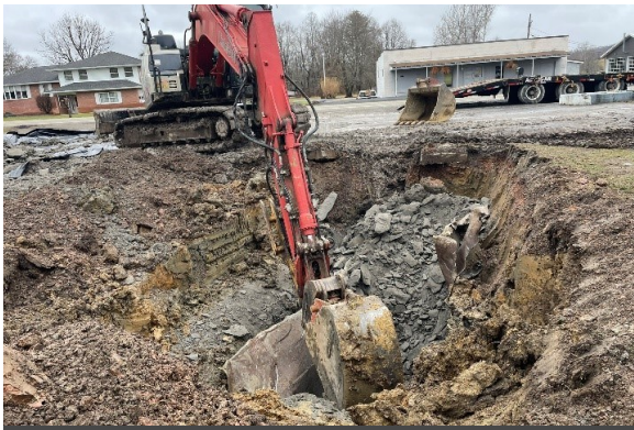
Heavy machinery breaking down and removing concrete-filled USTs.
