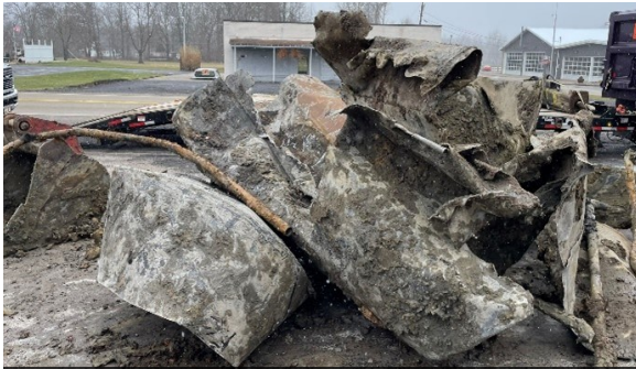
Several removed USTs are salvaged and processed for recycling.
