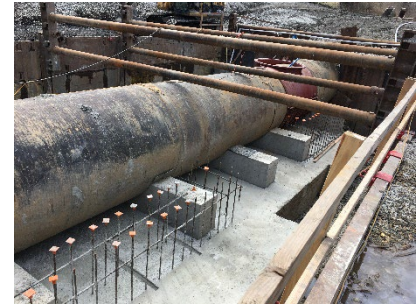
Photo credit: New Castle County
