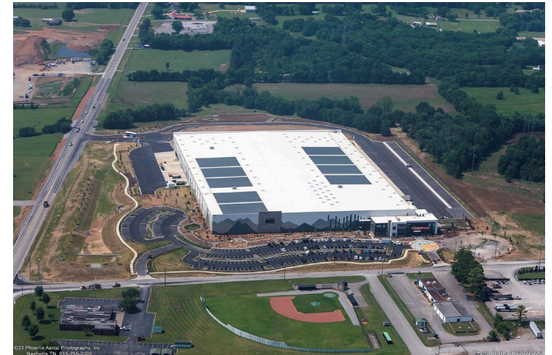
Aerial photo of rooftop solar on REI's newest distribution center in TN
