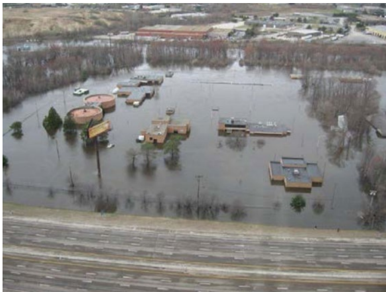
Figure 1: The flooded Warwick wastewater facility on Wednesday, March 31, 2010. (State of Rhode Island)
