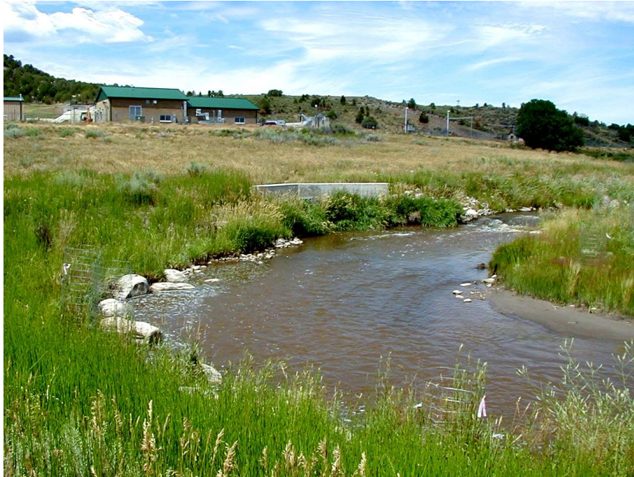
Figure 3. Outfall 002 to Rock Creek (Facility in background)
