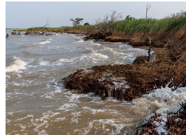
Storm/Flood Protection Erosion Protection
