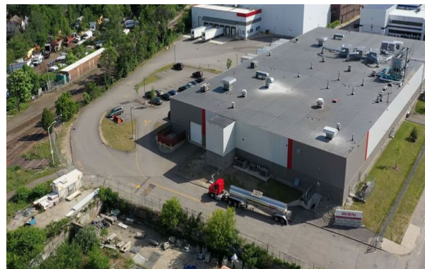
Aerial view of newly redeveloped 25 Southgate Street Facility. (Photo credit: Chacharone Properties)
