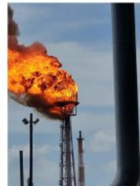
Air pollution from an improperly operated flare
