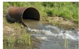
Discharge from NPDES outfall
