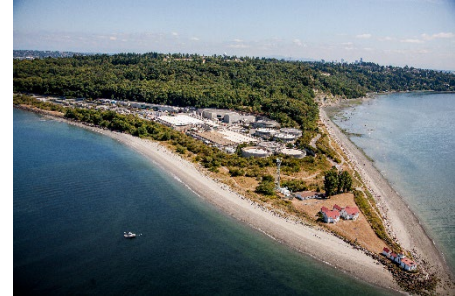
West Point Treatment Plant Photo credit: King County, WA
