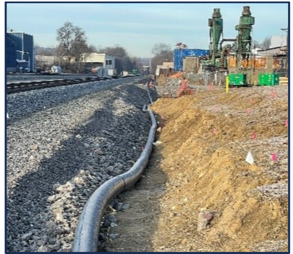
Photo 2 shows a view of the North Ditch bypass.
