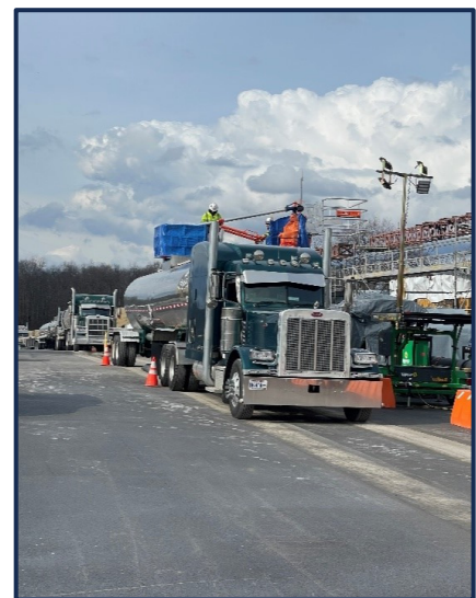
Photo 4 shows trucks being loaded with non-hazardous water for off-site disposal.
