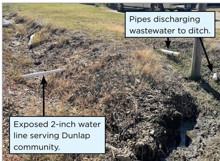
**Figures 3 and 4. Exposed water lines in Dunlap.**
