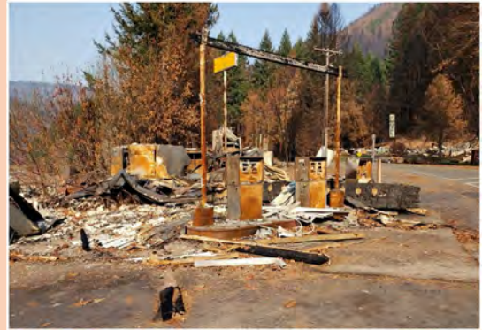
The Rivers Run facility after it was destroyed by the Lionshead fire
