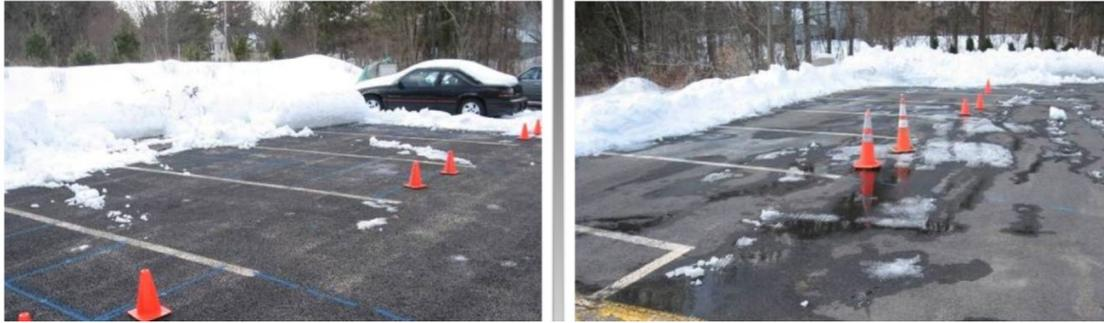
*Accumulation of standing water in a parking lot after snow melt. Comparison between porous pavement (left) and regular pavement (right). Source: UNH Stormwater Center*
