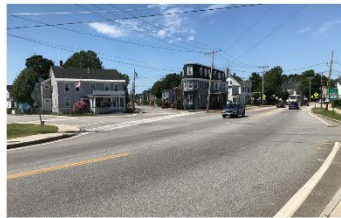
Figure 5: Current condition of North Main Street just west of the Cocheco bridge, facing west.
