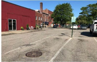
Figure 12: Current condition of public parking lot behind North Main Street businesses.
