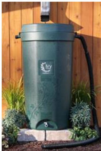
A rain barrel used to collect rooftop runoff using a gutter downspout system.
