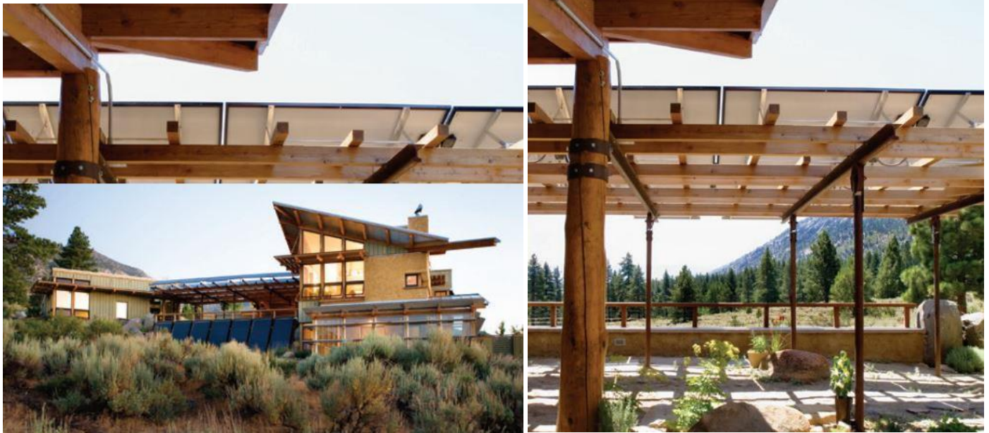
The Eastern Sierra House in Nevada was built with reclaimed wood and used airplane flaps were repurposed as garden shades. Photo: Edward Caldwell, Public Architecture Reuse Primer
