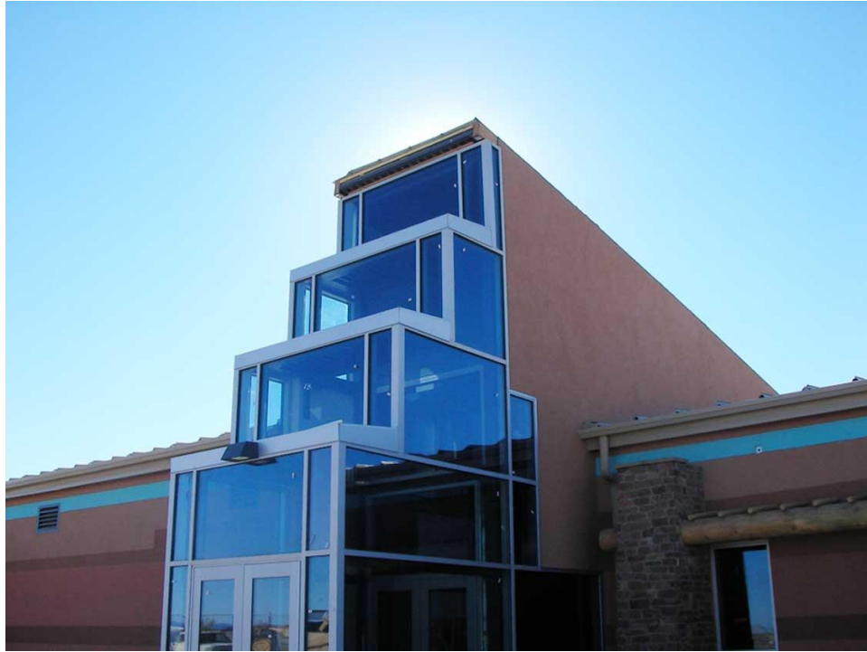
Kayenta Township, Arizona: Northeast Arizona Technical Institute for Vocational Education. Photo: Kayenta Township Building Department, 2011
