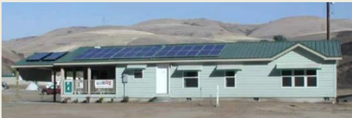
Zero Energy Manufactured Home, Nez Perce Fish Hatchery in Idaho. Photo: Washington State University Energy Program
