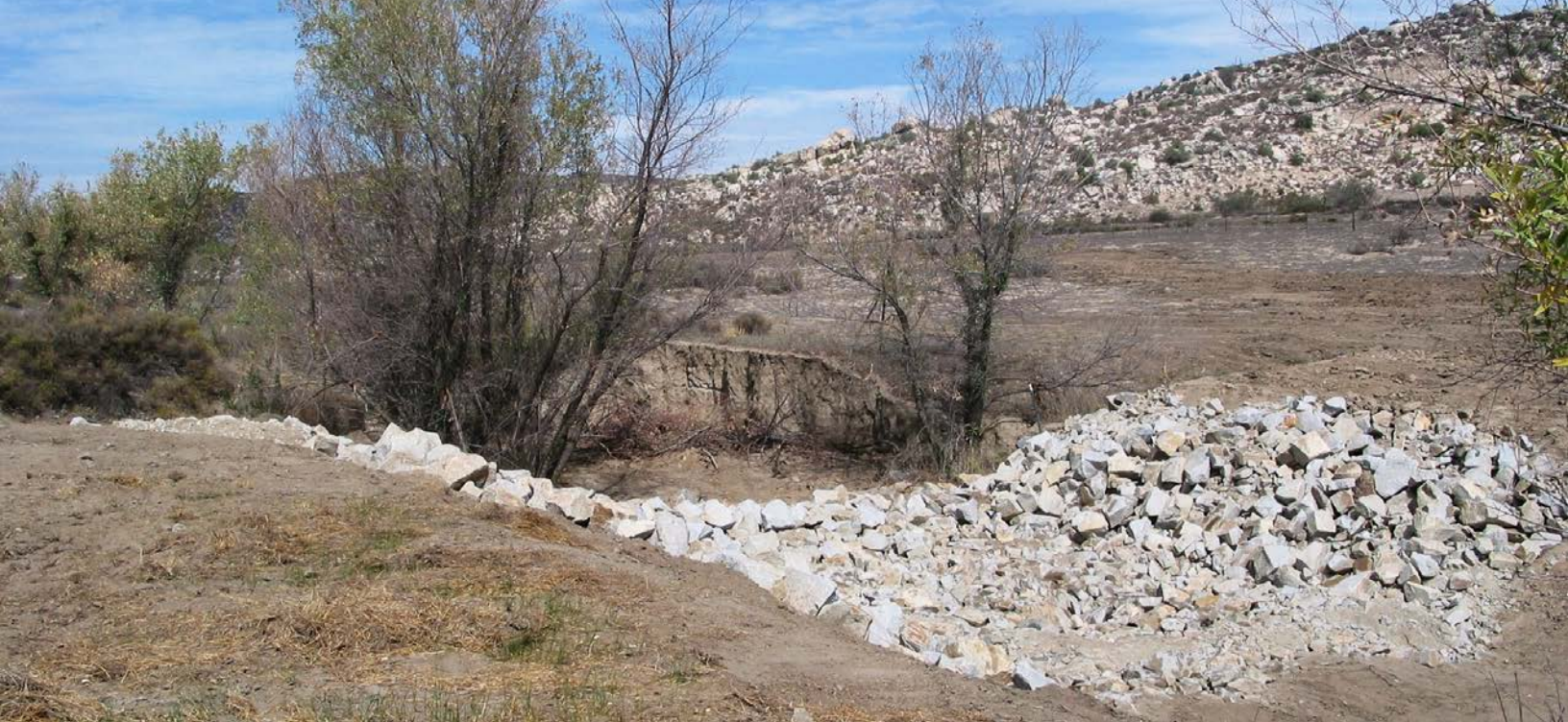
Diabold Creek detention structures that follow traditional Kumeyaay practices on the Campo Indian Reservation in San Diego County in 2002. Photo credit: Paul Ganster
