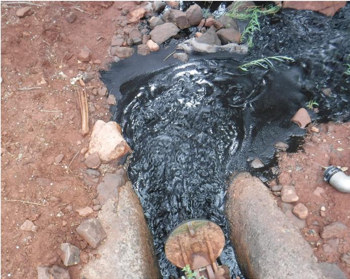
Fig 1: Manganese contaminants leaving a water system following ice pigging.
