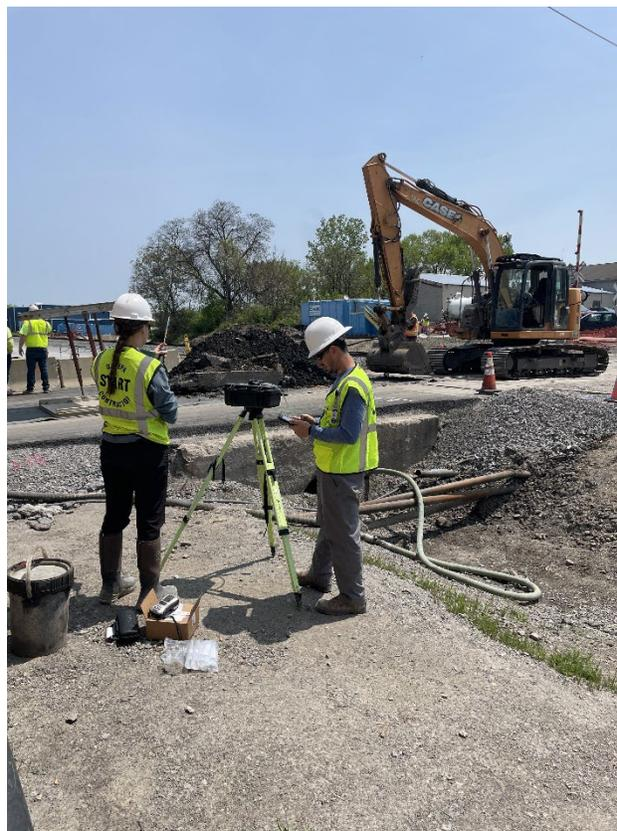
*Figure 4. EPA contractors checking on air monitoring stations. EPA has built and manages an extensive air monitoring and sampling network that uses several different technologies and approaches to provide separate and redundant sources of data on air quality at the derailment site and throughout the area.*
