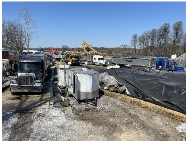
*Figure 7. Trucks being loaded with contaminated soil for disposal. More than 165,000 tons of contaminated soil and more than 35 million gallons of contaminated liquid have been shipped offsite for disposal.*
