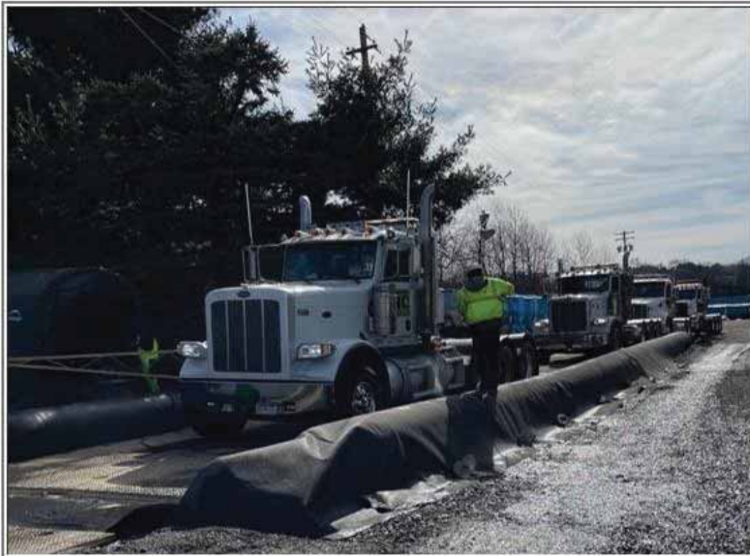
Trucks are pressure washed prior to transporting waste from the site.
