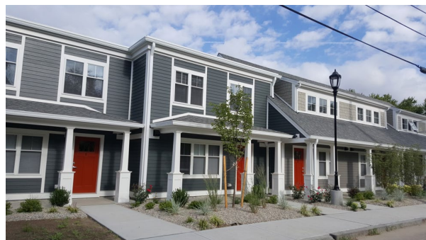
Affordable housing units completed in 2017 with support from EPA Brownfields grants (Photo Credit: Pawtucket Central Falls Development)
