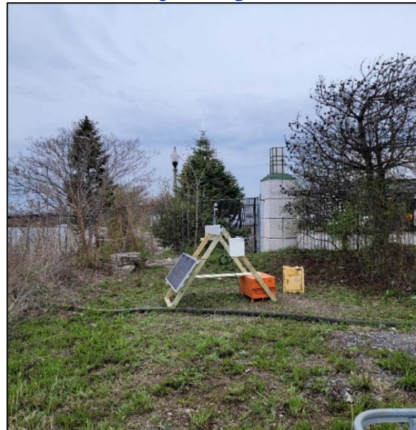
AQ5 Facing West
