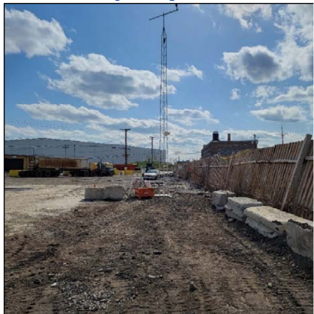
AQ1 Facing West
