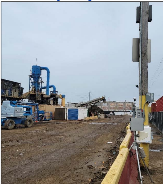
AQ3 Facing South
