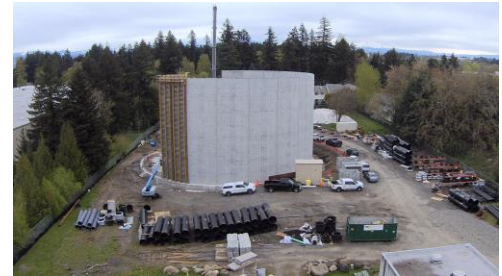
Photo credit: Rockwood Water People's Utility District
