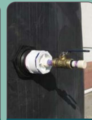
Trickle drain to ensure passive function
