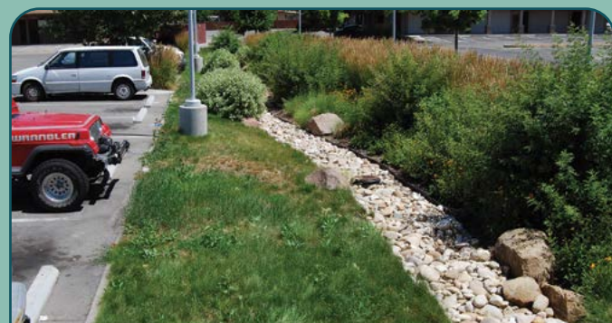
In this library parking lot an irrigated bioretention system has been incorporated into a wide parking lot island. Note the stone channel used to distribute runoff throughout the bed.
