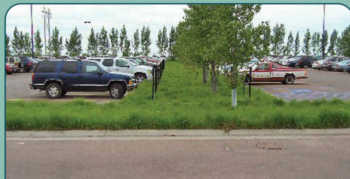
Bioretention can be integrated into parking lots such as this example of a grassed bioretention area in Fargo, ND.
