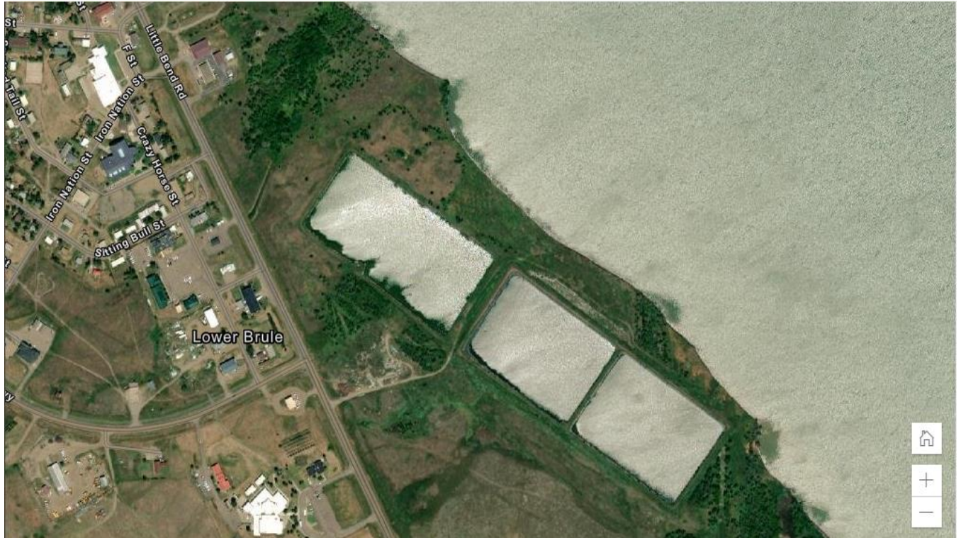
Figure 1. Lower Brule Lagoon System Aerial a/
