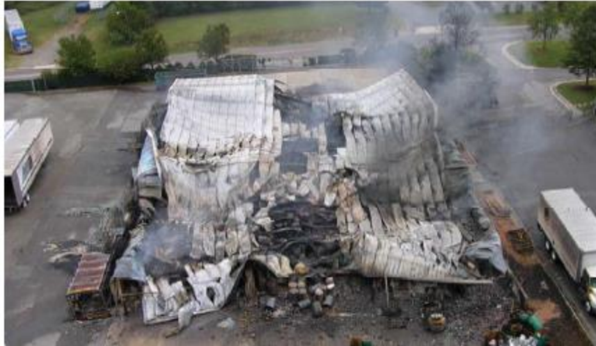
Photo: Wake County Fire/Rescue Services.
