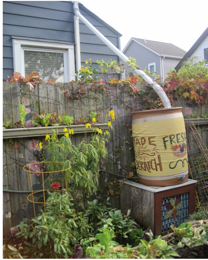
A rain barrel decorated by a homeowner and used for watering a garden. Credit: Alisha Goldstein, USEPA
