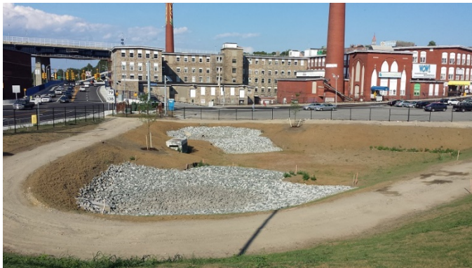
Infiltration basin in an urban area. The basin has two gravel areas for infiltration. The remainder of the basin bottom and its slopes are planted with sod.
