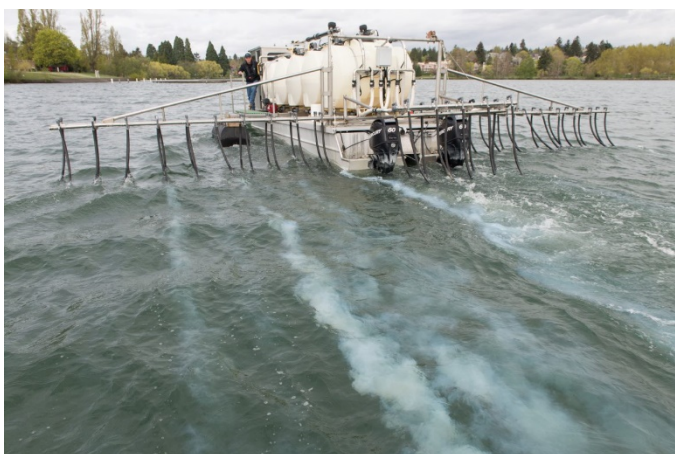
A barge fitted with specialized equipment (tanks and distribution lines) can evenly distribute alum in large surface water bodies.
