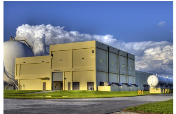
Central District Wastewater Treatment Plant Credit: Miami-Dade Water and Sewer Department
