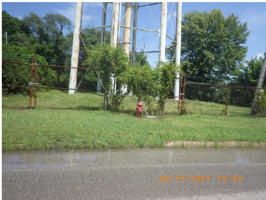
RIMG1471 Ongoing flushing in Cahokia Heights near the water tower near Church St. and S 57 th , 8/11/21
