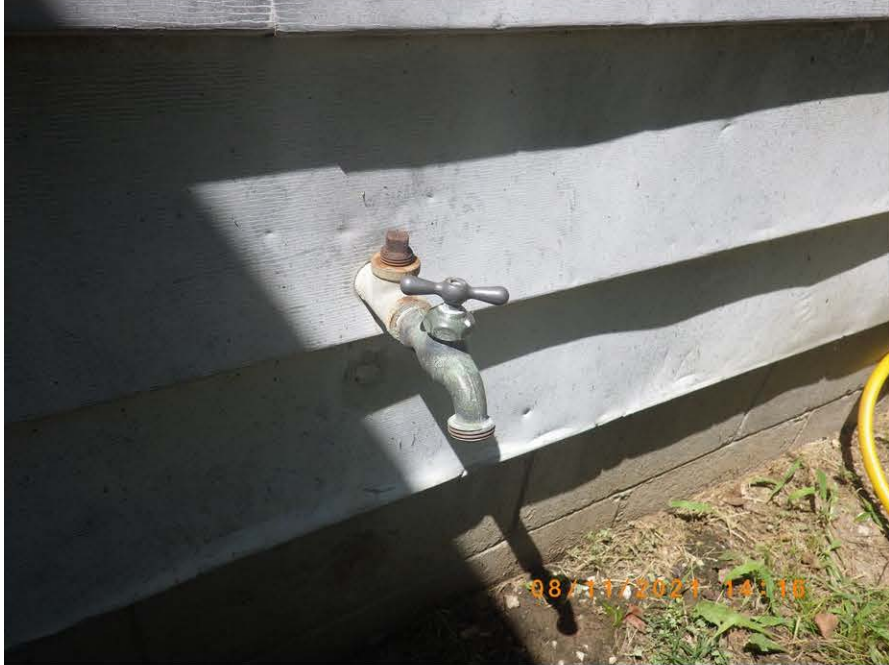
RIMG1472 Hose bib at site 1-09, 5603 Old missouri Ave, 8/11/21
