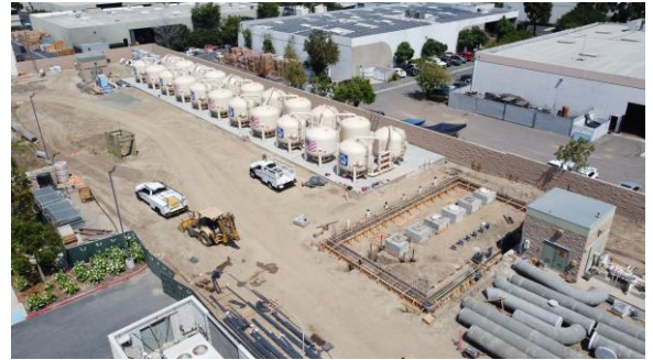
Photo credit: Orange County Water District
