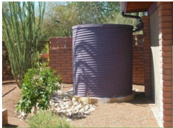
Rainwater harvest demonstration
