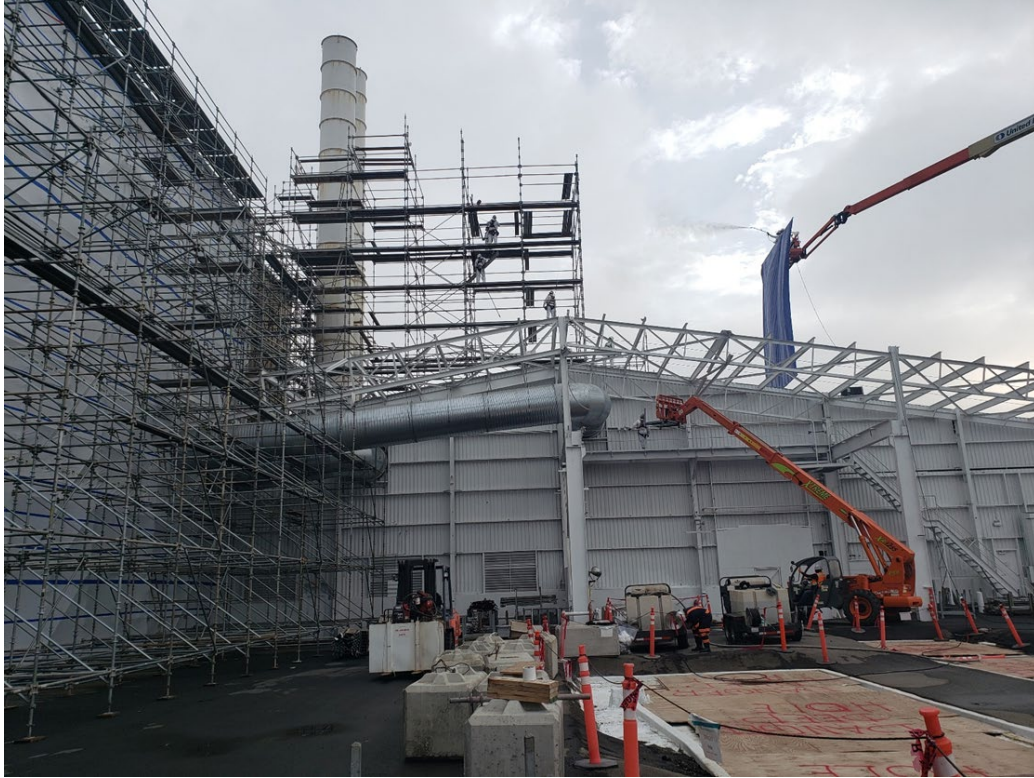
Remaining FEU 2 Scaffolding Dismantlement with Enhanced Dust Suppression (6/18/21)
