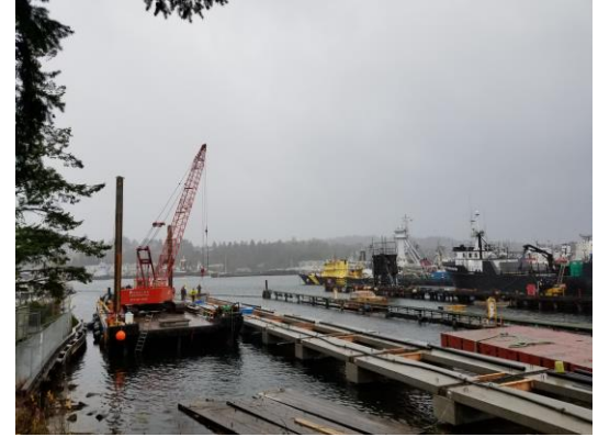
Seattle Project Construction
