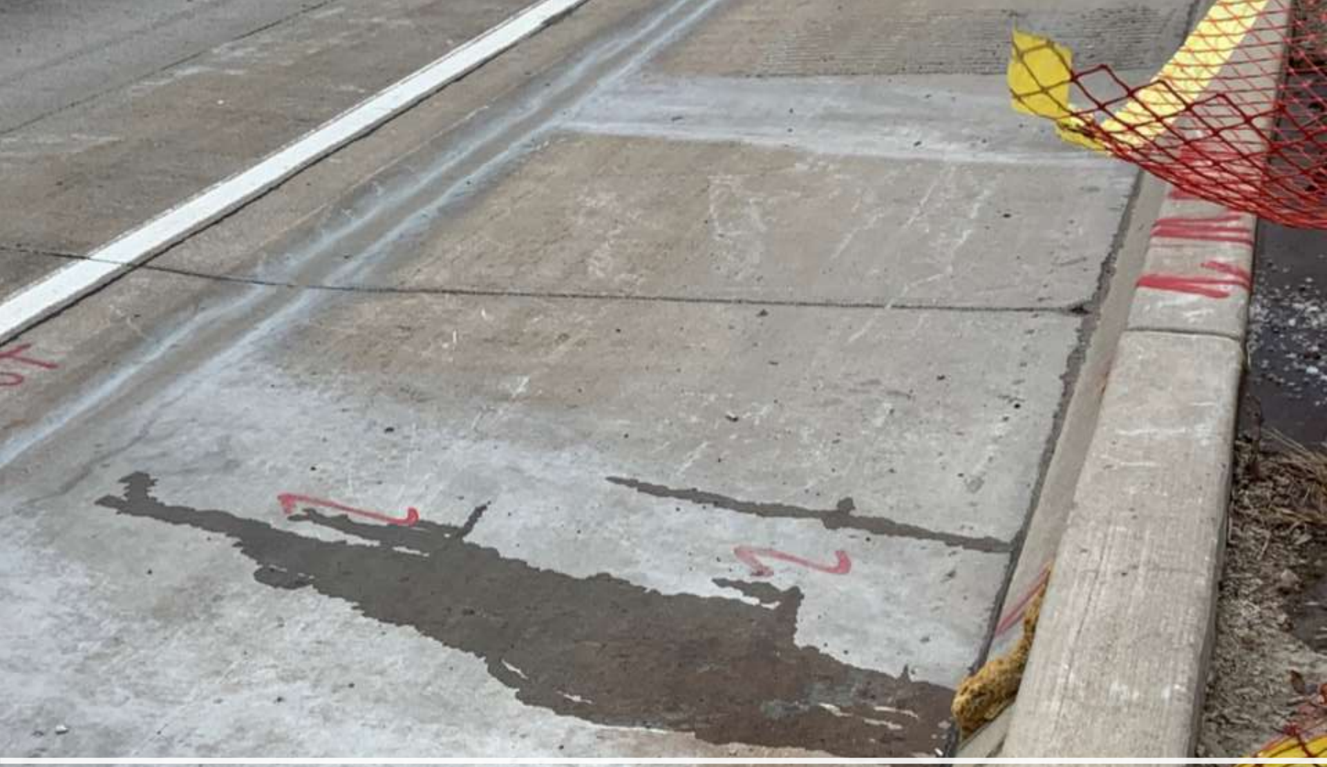
I-696 Embankment Wall
