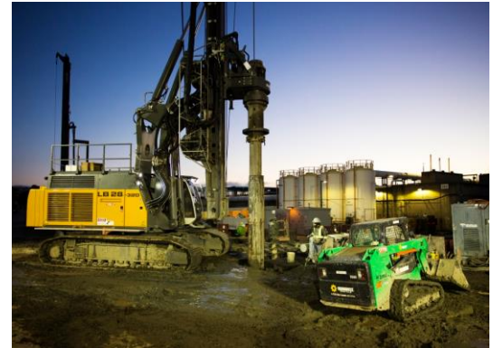
Construction on Treatment Facility
