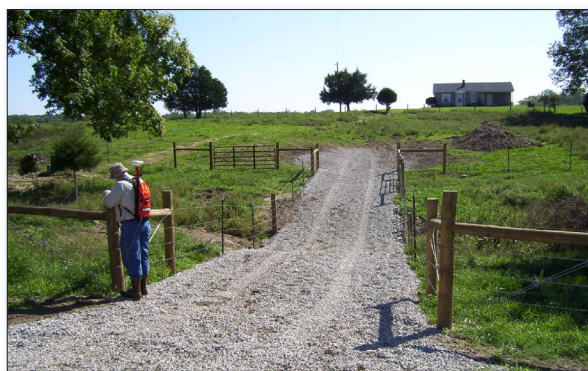
Figure 2. This stream crossing prevents cows from accessing the creek.
