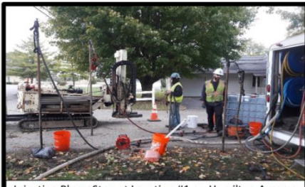
Injecting PlumeStop at Location #1 on Hamilton Avenue
