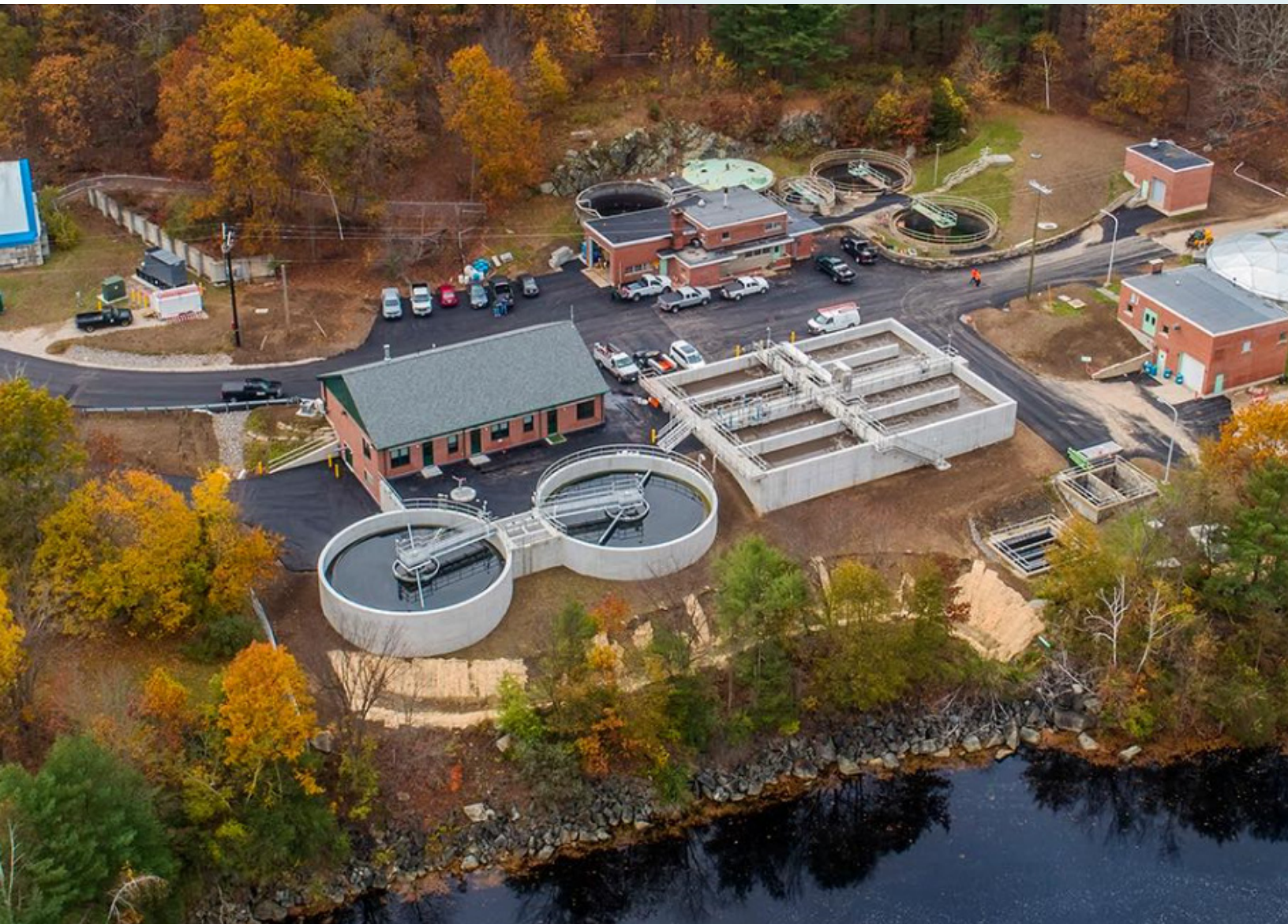
2019 New Hampshire PISCES Project: Town of Newmarket Wastewater Treatment Facility Upgrade
