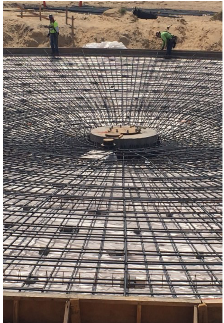
AIS Site Visit: Water Reclamation Facility Expansion Project, Apopka, FL
