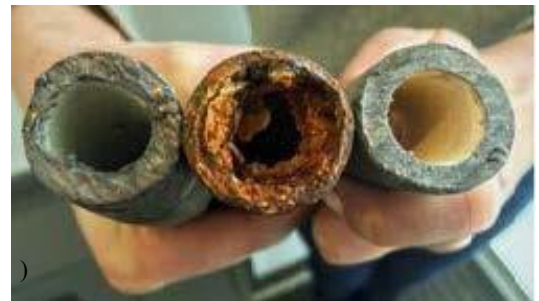
Lead service lines showing inner surface without any coating from corrosion control treatment (left), with coating (right), and fully corroded (middle). (EPA photo)
