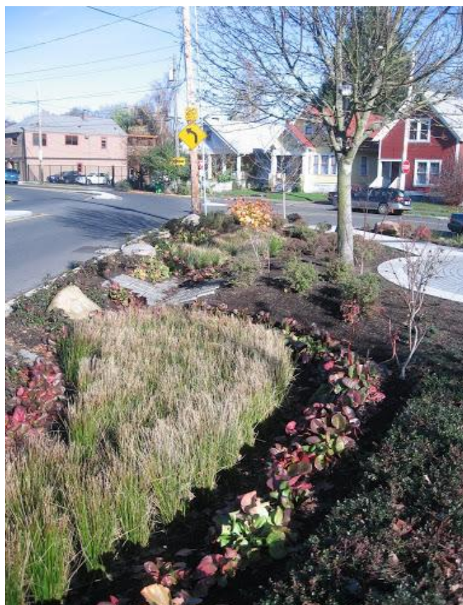
Curbside rain garden installation in Portland, Oregon.
