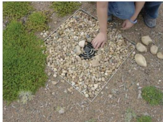
*Image 31.1. Vegetation free zone around roof drain being cleaned out. Photo courtesy: Urban Drainage and Flood Control District.*
