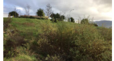
This 300-yard-long bioswale on the Santa Ynez Reservation in California is designed to reduce flooding danger to surrounding homes. It also provides wildlife habitat.
