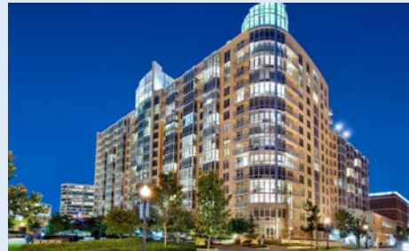
A 75-kW system provides electricity and hot water at the Wisconsin Place Apartments (above) and a 150 kW system powers the 4701 Willard Apartments (below).
