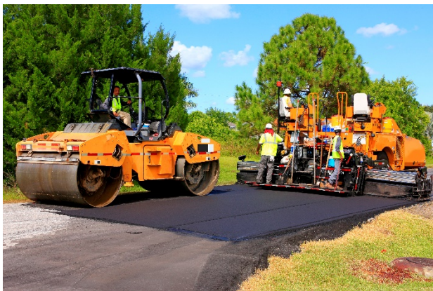
Road resurfacing that does not disturb the subsurface.
