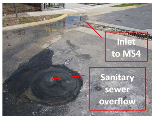
Wastewater flowing from a sanitary sewer access manhole to a nearby storm drain system inlet. Photo: PG Environmental
